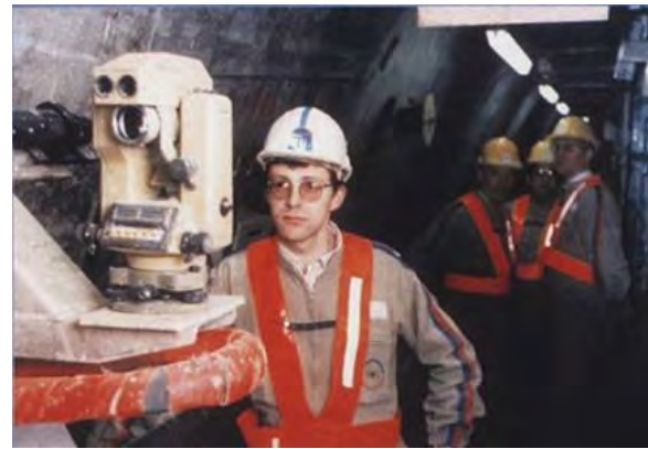
Above: Direction control of the tunnelling machine in the Channel Tunnel in 1987 with Wild T1600 electronic theodolite and Wild DI3 infrared laser distance meter from Heerbrugg.
