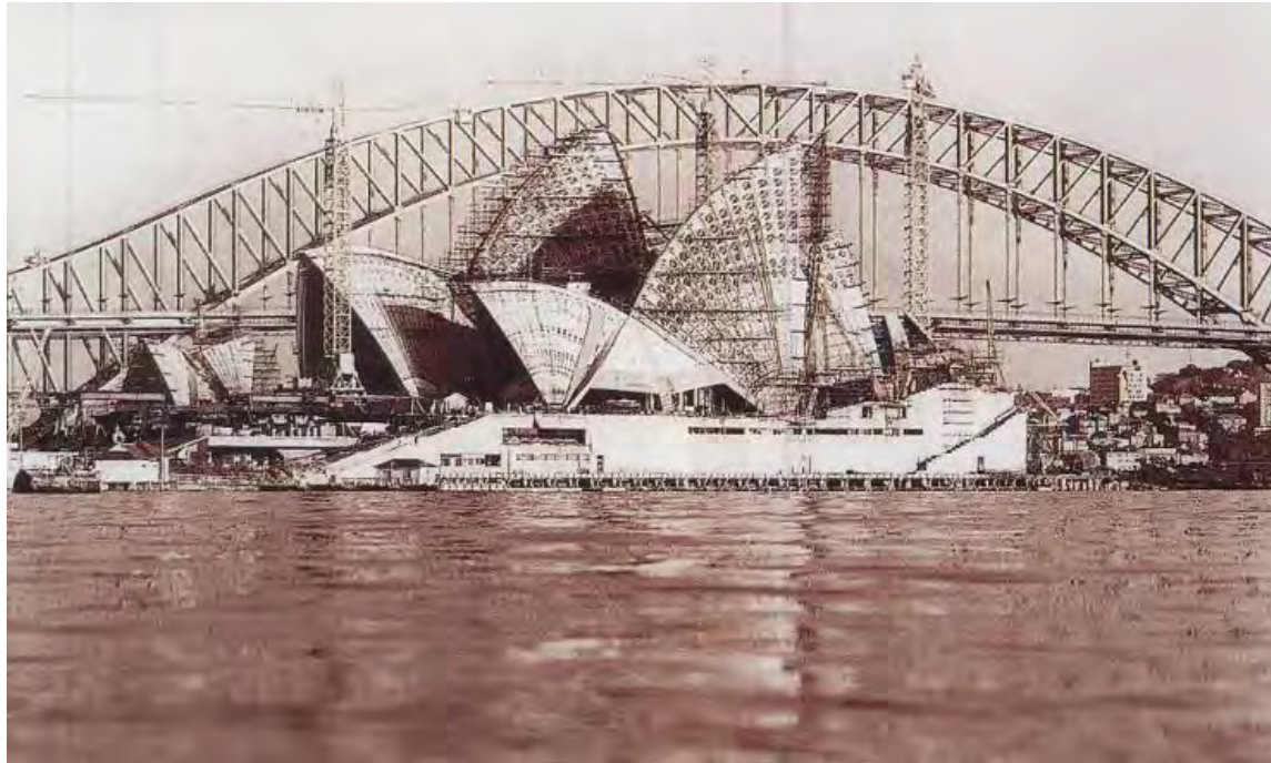
Construction of the Sydney Opera House in 1968 with Wild T2 and Wild DI10 IR laser distance meter / reduction tacheometre,
